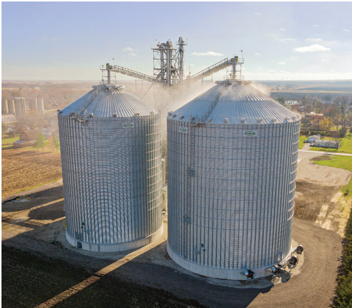
*Standard roof peak loads meet ASCE 7-10 for unbalanced snow load with 40 psf ground snow load.
